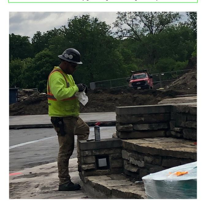
Propane is secured and maintained at least 10 feet from burners
